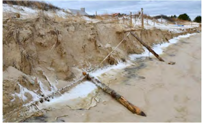
Example of symbolic fencing damage on an erosive beach. To avoid this result, fencing will not be placed near the sand trap.
